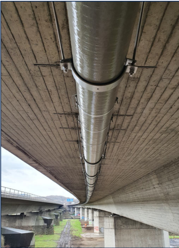
A3, Ruhrbrücke, Duisburg
